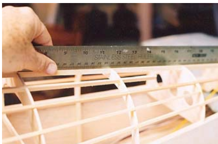
23. Check stringers with a straight edge while and after glueing in place.
